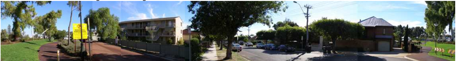
Carr Place cul-de-sac turning head frontage
