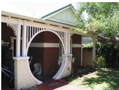
Figure 15: Heritage site. No. 40 Anzac Road, Mount Hawthorn
