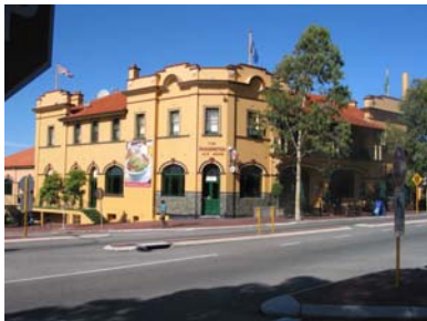
Figure 13: Heritage site. No. 141 SBR, Mount Hawthorn
