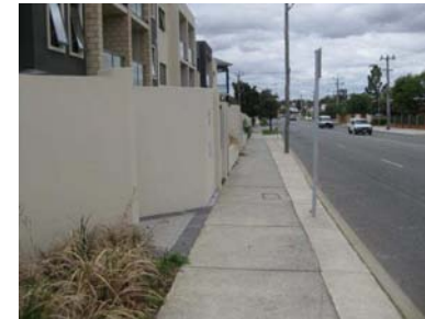
Figure 5: Heading eastward, bad pedestrian/cycling environment along this portion of SBR, as there is no buffer between the footpath and traffic
