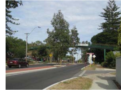
Figure 3: Overhead pedestrian bridge between Braithwaite Park and the school
