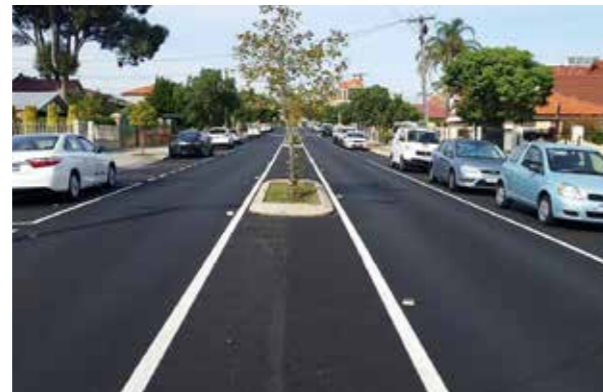
A recently resurfaced road (Angove Street - District Distributor B)
