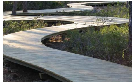
Figure 54. Example of raised timber boardwalk.
