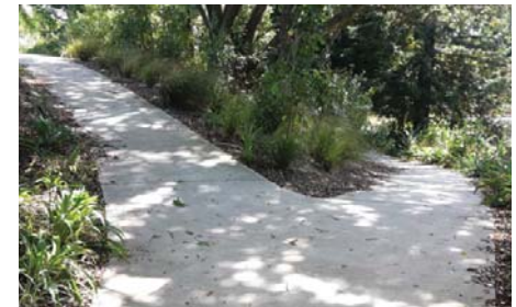
Figure 50. Sloped paving treatment.
