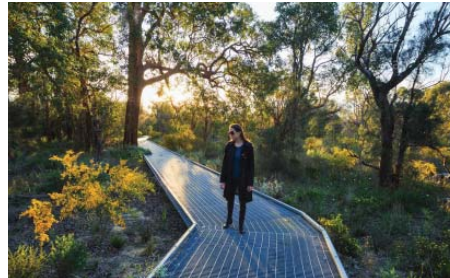
Figure 55. Raised perforated steel boardwalk.
