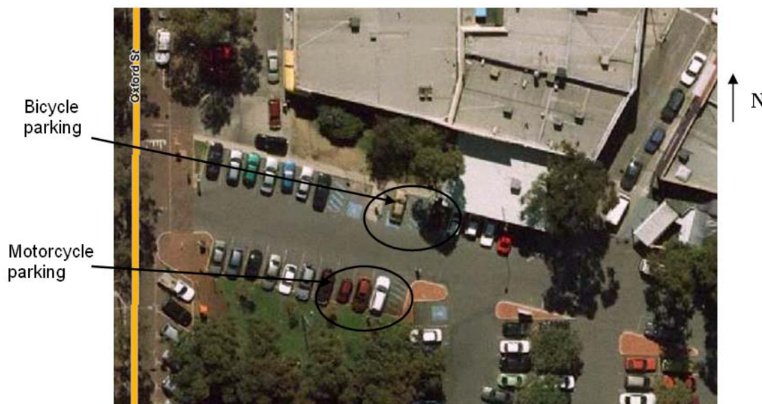
Figure 3: Provision for motorcycle bays in Frame Court
