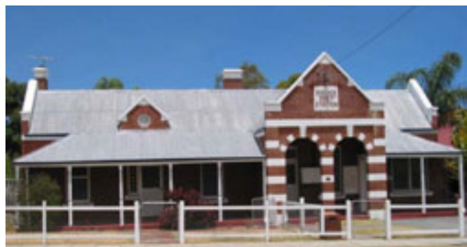
On the cover and above: Built in 1907 and designed by Hillson Beasley in the Federation Free Classical style, the former North Perth Police Station in Angove Street was purchased by the Town for use as a community facility.
