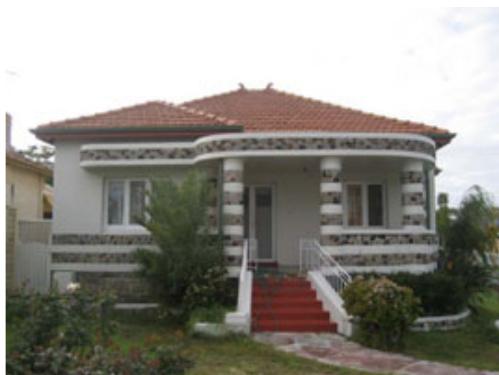
The Heritage Assistance Fund provides funding for works on heritage-listed properties. This Post-War Immigrant Nostalgic Bungalow's fascias, gutters and down pipes were replaced and the render re-painted.
