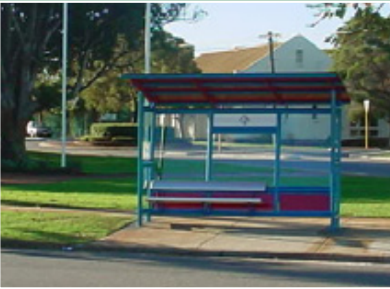
Four new bus shelters were installed during the year.
