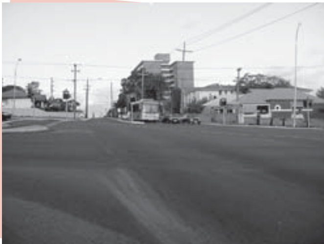
State Black Spot program: New slip lane at the intersection of Vincent and Loftus Streets, North Perth.
