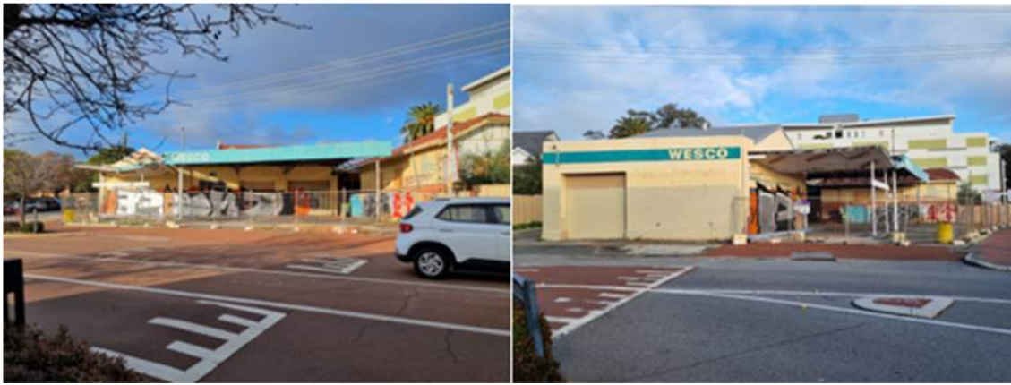
Figure 1 – Existing Site Conditions – Angove Street (L) and Woodville Street (R)
