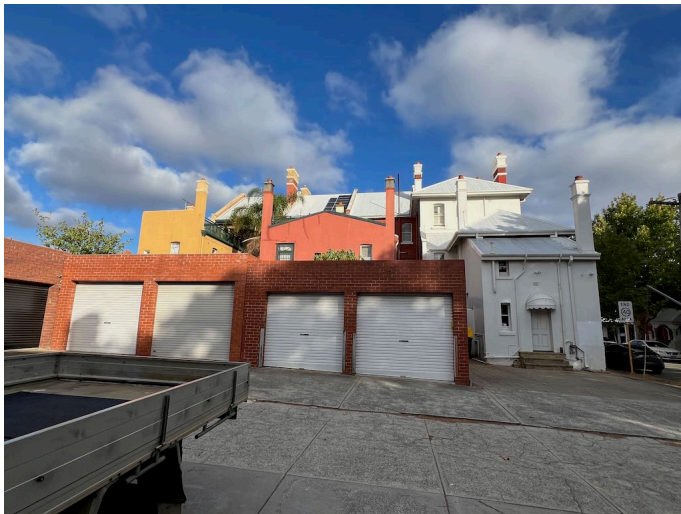
View to southeast from the rear of 56 Lindsay Street showing the rear of the Beaufort Street buildings and garages.
