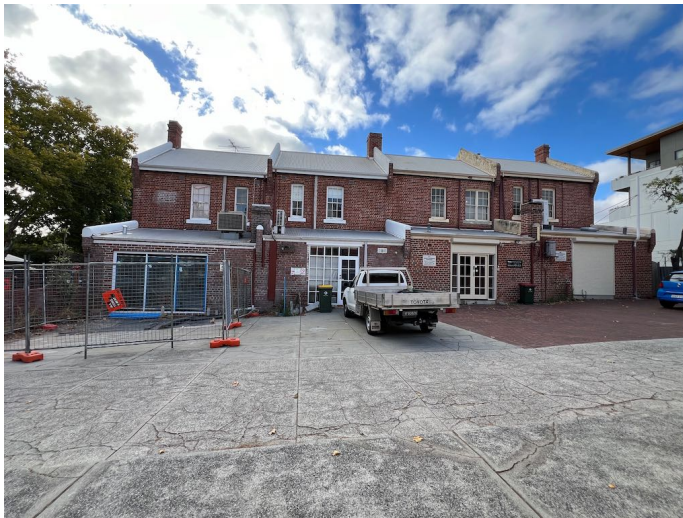
Rear (southeast) elevations of the terraces (No. 56 with vehicle).
