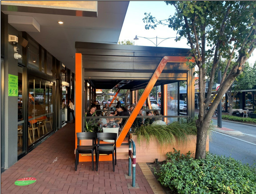
PHOTOGRAPH 26: 5:59pm. The blind is retracted as the sun is no longer filtering into the alfresco area at a level which concerns the customers. The space is activated, visually permeable and continues to add vibrancy to this public space.
