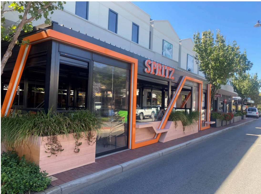
Figure 1 – Alfresco Structure from the south & with a section of clear blinds in use
