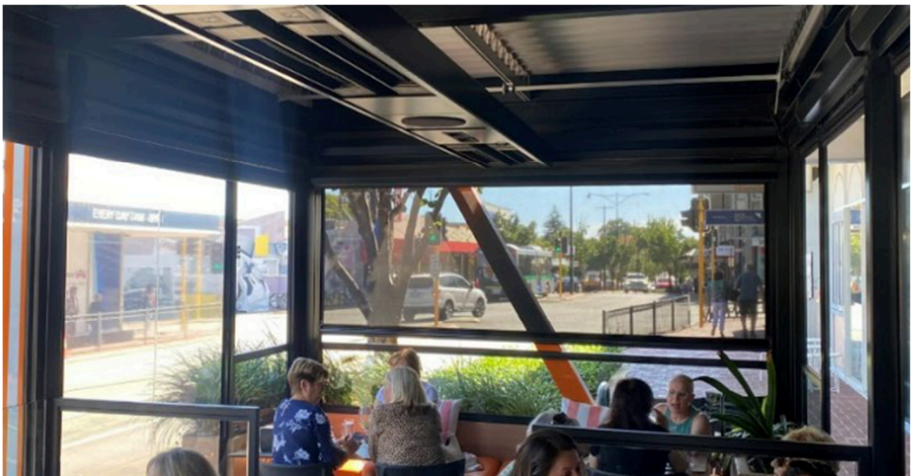
Figure 3 – Internal view facing west, showing clear plastic blinds and woven mesh blinds in use
