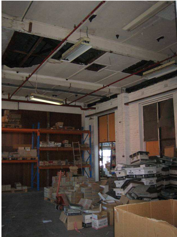
Interior portion of structure along Pier Street
