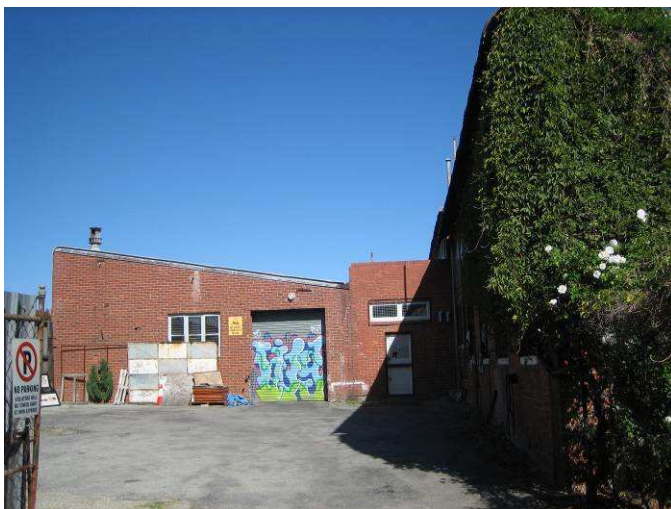
Southern portion of the East facing elevation
