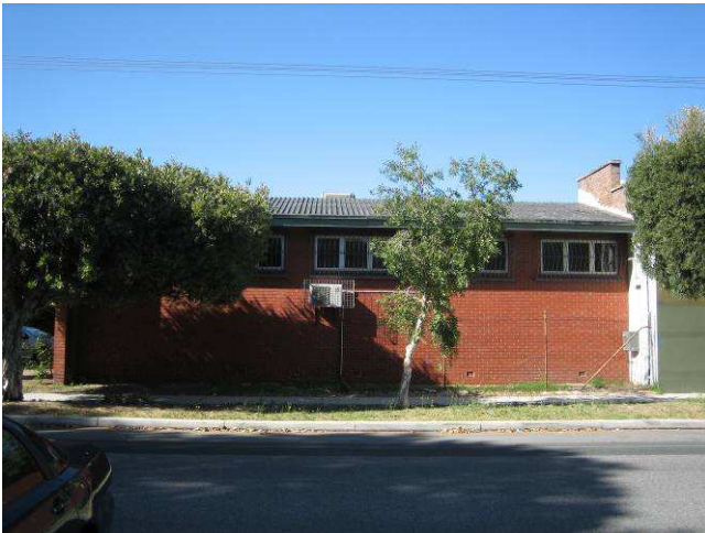
North facing elevation (far eastern end)
