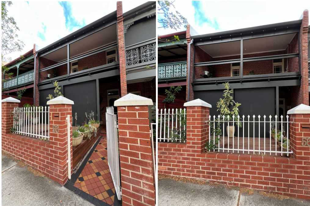
Front views of the 56 Lindsay Street terrace. (original balustrade infill is offsite being restored).
