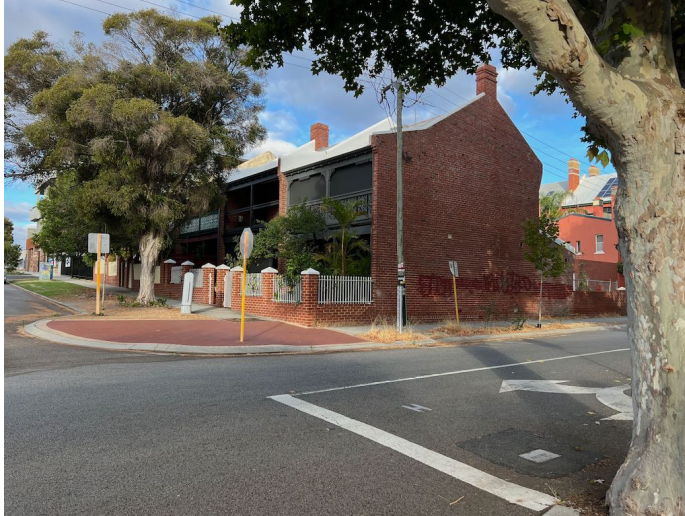
Streetscape view looking east from the Lindsay/Money streets intersection.
