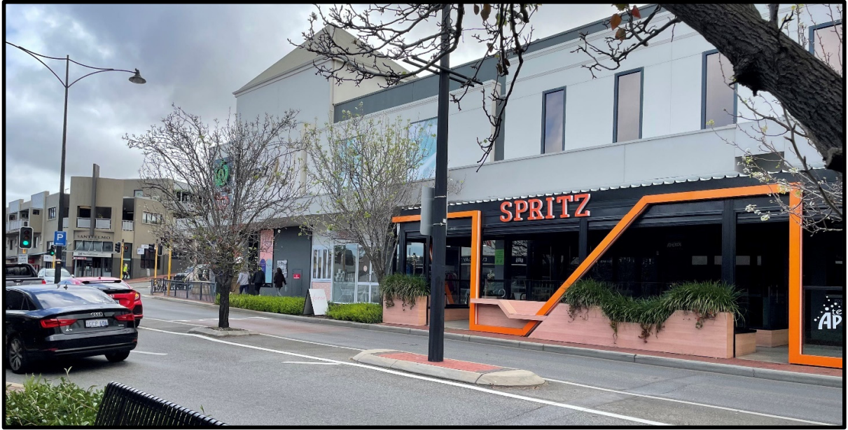
Photograph 3: Standing on the southwestern side of Scarborough Beach Road looking towards the canopy structure. Note: the design retains visibility and accessibility through the space, inviting pedestrian movement through and within it.
