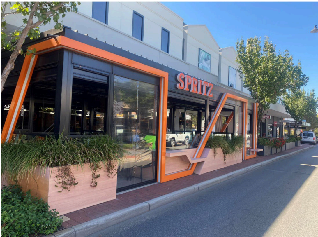
Figure 1 – Alfresco Structure from the south & with a section of clear blinds in use
