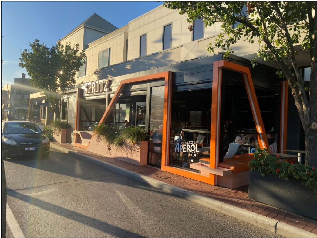
PHOTOGRAPH 20: 5:21pm. The mesh blinds are not in use as it is not necessary.
