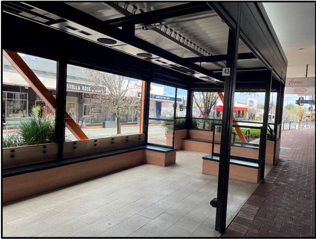
Photograph 4: Standing on the northeastern side of Scarborough Beach Road in the pedestrian footpath clear zone between the alfresco dining area and the internal dining area of the restaurant. Note: The tables and chairs are removed from the space and the motorised blinds are retracted, as Spritz was not open for trade when the photograph was taken and the weather conditions at this time of the day did not require the blind system to be activated to shelter the space. This space is available to the community to use when the restaurant is not open.
