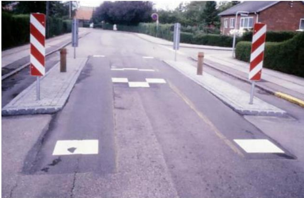
Figure 8.3: Combination road hump (Copenhagen)
