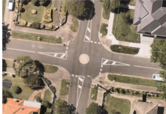
Figure 2: a typical mini roundabout in metropolitan Melbourne, Victoria
