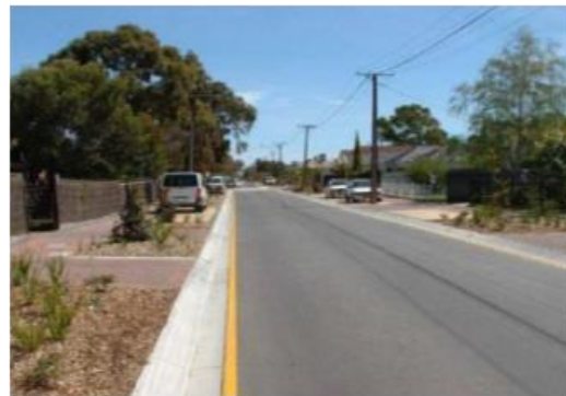
City of Mitcham, South Australia
